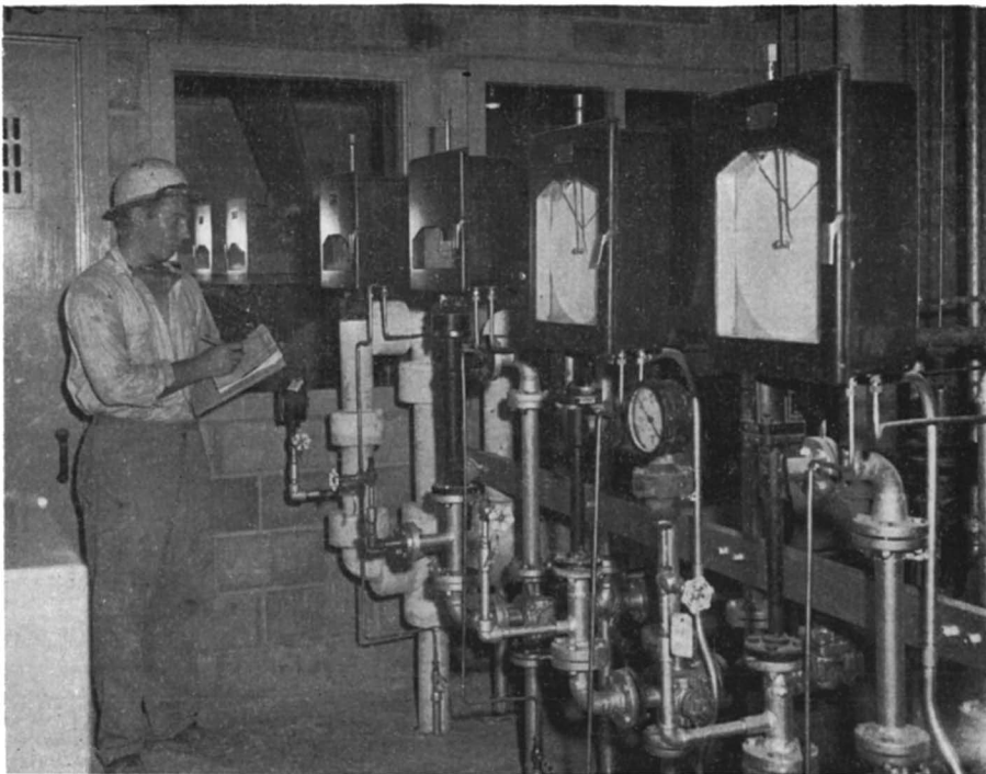
Operator checks 24-hour recording charts showing flow of water, sulphuric acid, nitrogen solution and anhydrous ammonia into ammoniator. Control room is fully automatic.
