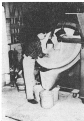
TVA Pilot Plant Pan Granulator
