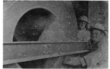
Slide 7 T.V.A. Ammoniator in operation
