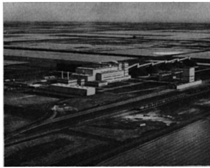
Figure 5 Overall Plant View
