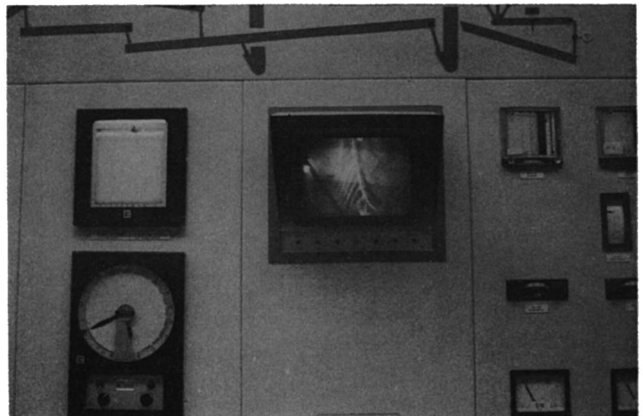
Figure 3 Part of control panel at Forenade (Sweden) NPK plant showing television view of granulator discharge.
