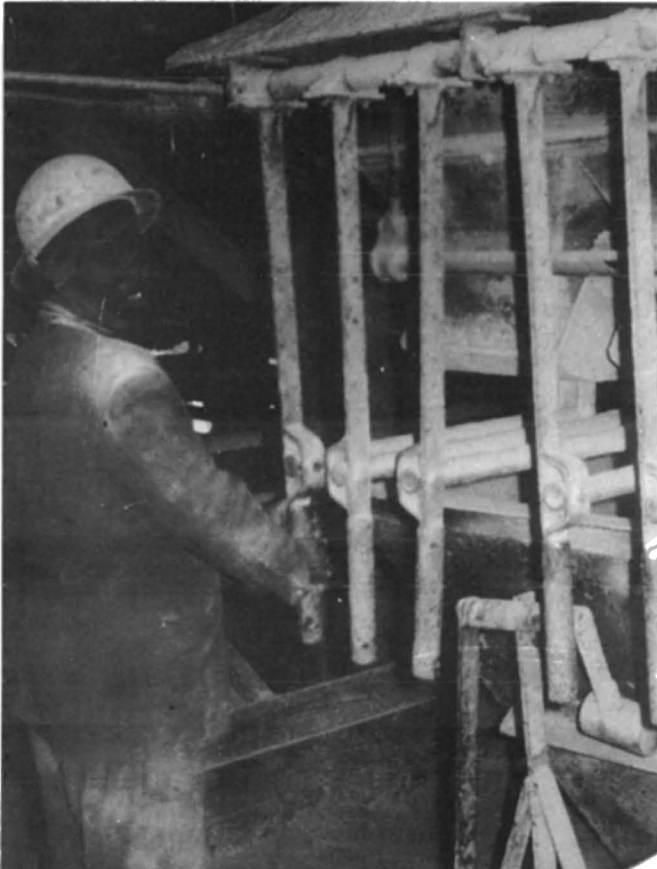
FIGURE 4. MATERIALS WEIGHED INTO HOPPER FROM 6-BIN OVERHEAD CLUSTER HOPPER SYSTEM
